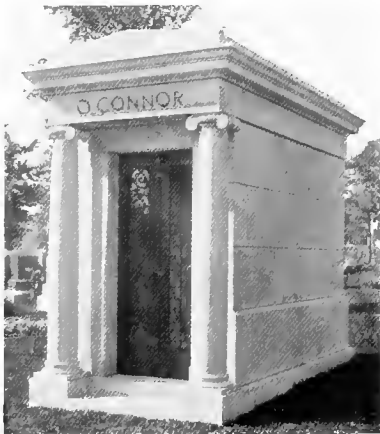
Number 8260. This attractively proportioned building contains three catacombs. Erected in Woodlawn Cemetery, New York.
